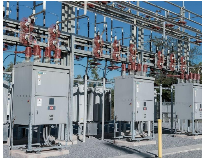
OUTDOOR MEDIUM VOLTAGE SWITCHGEAR
